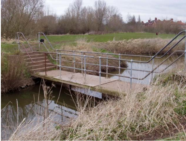
Photo: One of the old bridges
