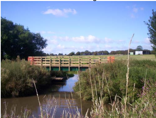
Photo: One of the new bridges
